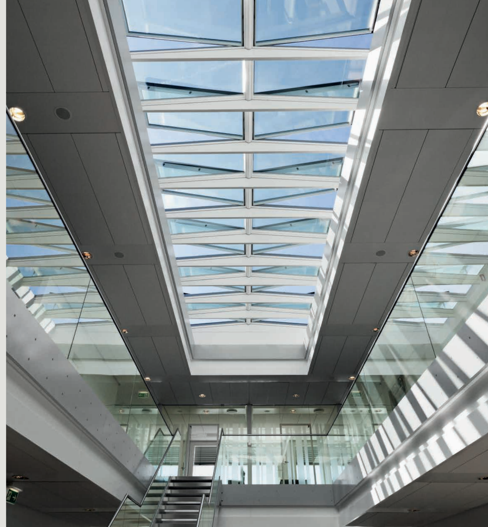
Ridgelight 5° in the ATP building, Vordingborg, Denmark – open modules.
