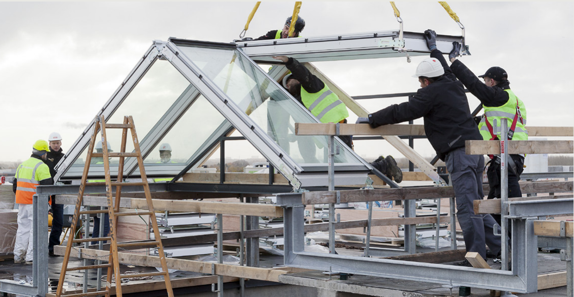
The modular skylights are lifted into place in the self-supporting ridgetlights by crane. The modules rest on steel profiles on either side.
