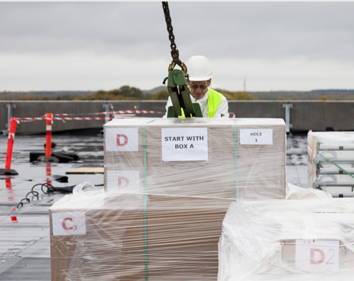
Master carpenter John Wulff receives the modular skylights as an assembly set, clearly marked with letters and numbers.
