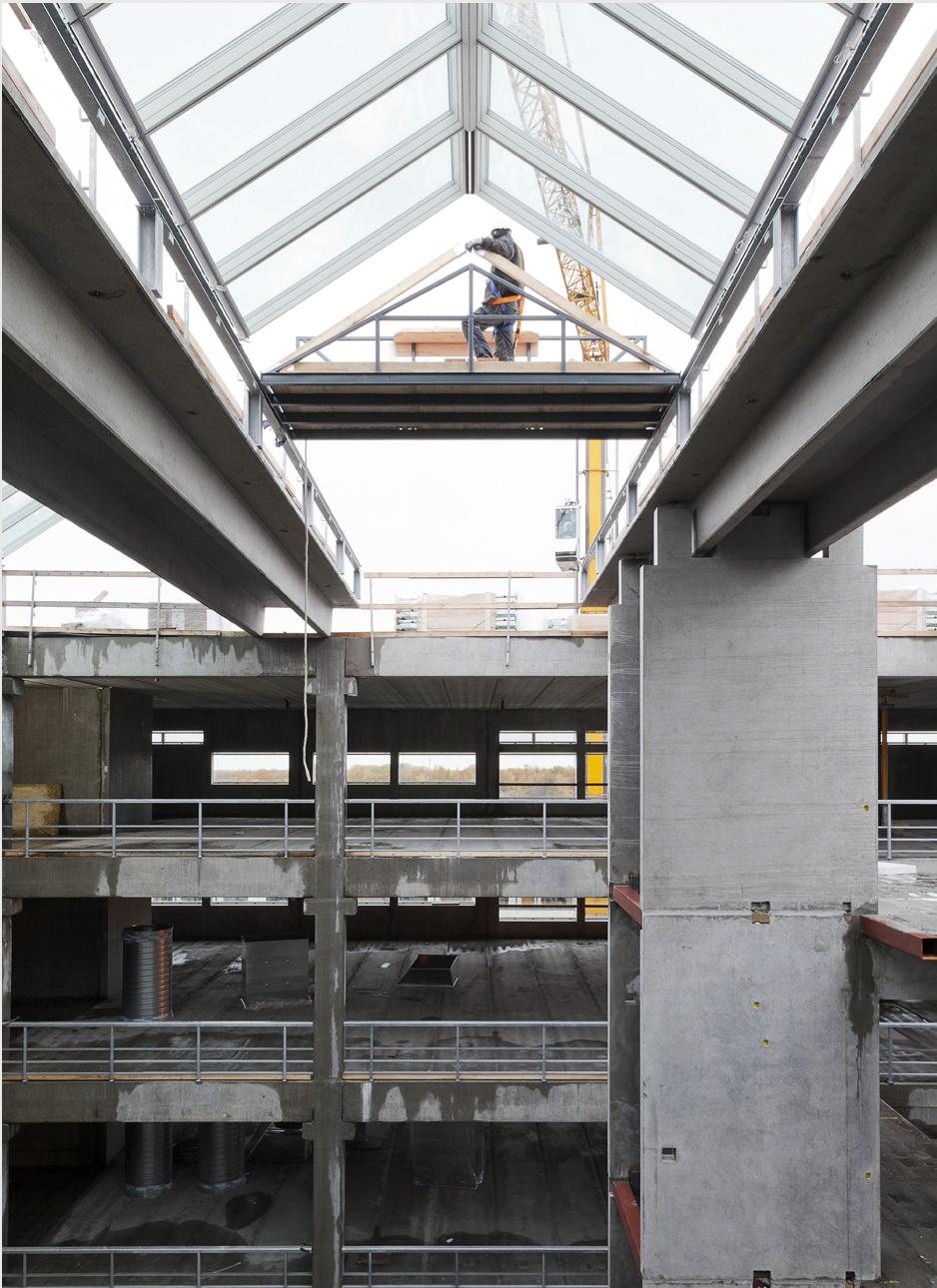
The modular skylights are assembled 25 metres above the ground using a rolling platform. According to John Wulff, it takes on average 7-8 minutes to install each modular skylight.
