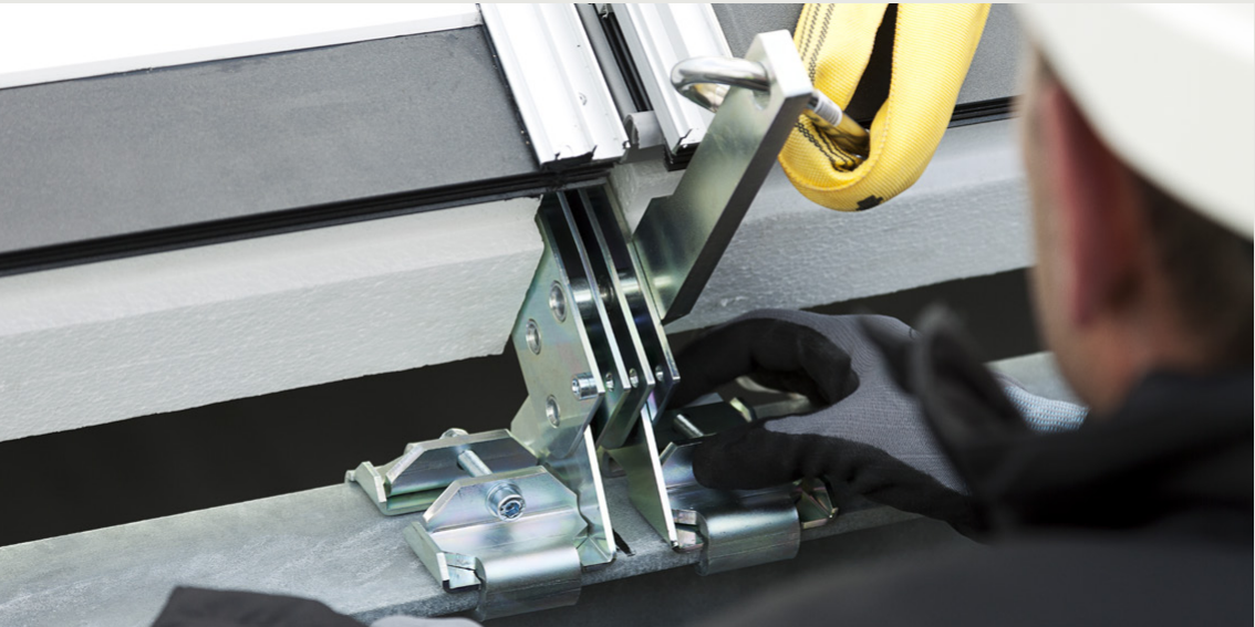
The modular skylights are fastened to the steel profiles with patented clamps.
