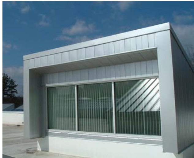
Figure 5. A close-up view of a roof monitor at Smith Middle School.
