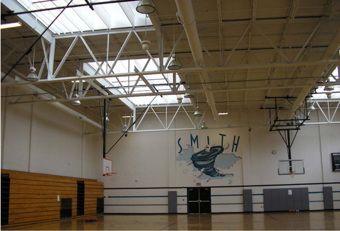
Figure 13. Roof monitors and baffles do an excellent job of daylighting the gymnasium at Smith Middle School.
