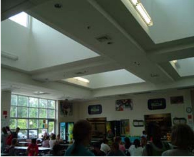
Figure 15. North facing roof monitors without baffles provide daylighting for the cafeteria at Smith Middle School.
