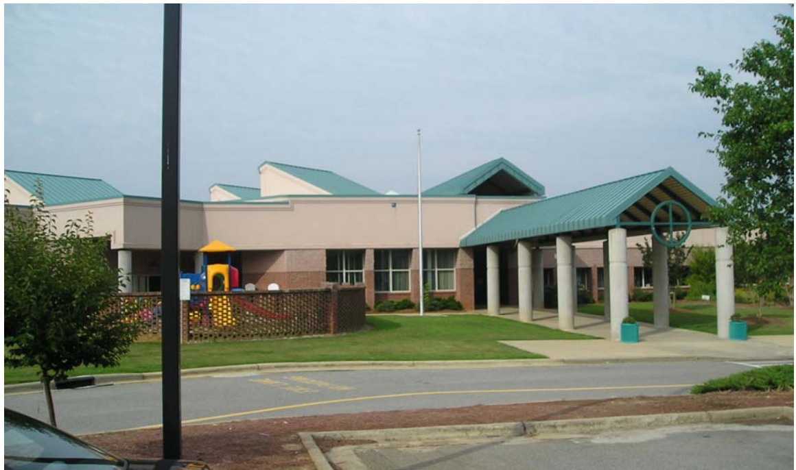
Figure 2. South facing roof monitors on flat roof at East Clayton Elementary School.
