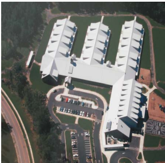
Figure 6. A top view shows the symmetrical arrangement of the raised dormers that create the clerestories at Rashkis Elementary.
