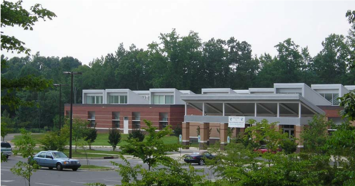
Figure 3. A front view of Smith Middle School. Note that all roof monitors are oriented south.
