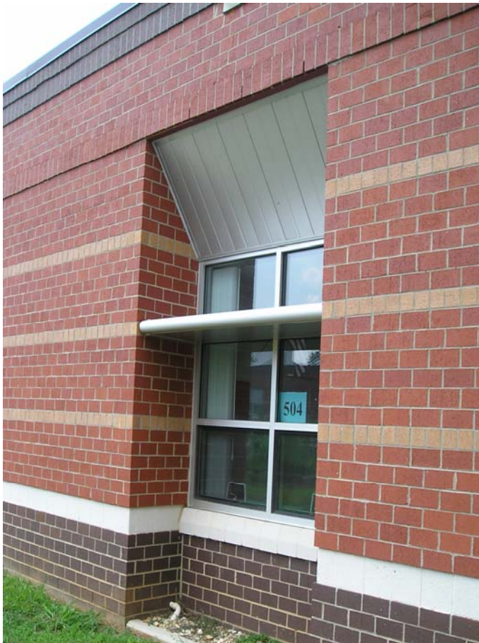
Figure 9. Most south facing windows at Smith Middle School are recessed approximately two feet. Note the anodized aluminum light shelf incorporated into the window arrangement.
