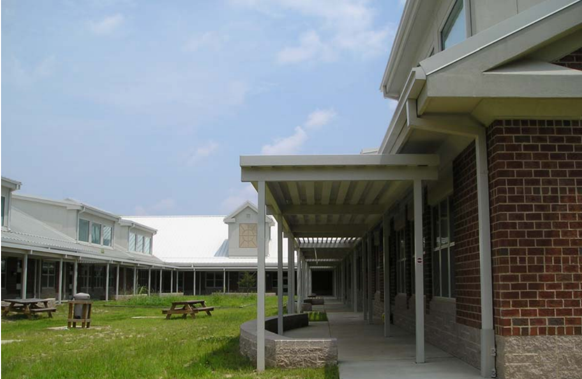
Figure 12. A close-up view of the covered walkway and its shading effect at Rashkis Elementary School.
