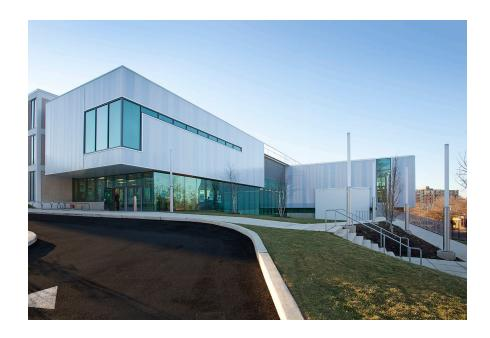
that eliminates the need for vulnerable wet seal and adhesives, the UniQuad is the only daylight system that can span as long as 12 ft. between structural supports. Scalable, the UniQuad can be configured with additional insulation, Class A fire-rated assembly, sound reduction, dynamic shading, additional structural performance and military forced entry resistance, always maintaining its integrity.
