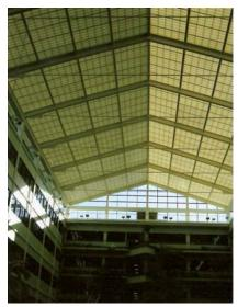
A discolored and deteriorated skylight (bottom photo) was replaced with a Quadwall system (photo above taken during removal and installation) resulting in a dramatically improved work environment with pleasant natural daylighting (top photo).
